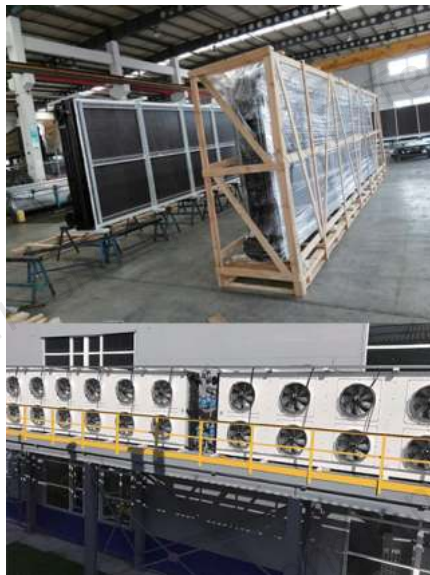
Country: Russia Application: ore yard cooling Cooling capacity: 493kW Cooling medium: 20% ethylene glycol Supply power: 400V/3P/50Hz Fan brand: Ziehl-Abegg
