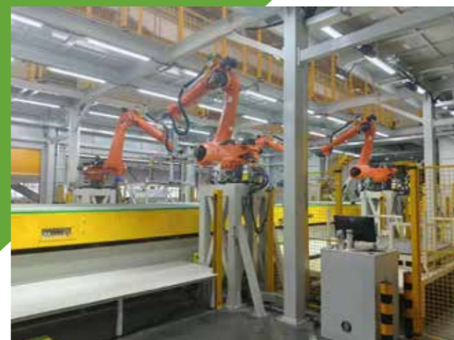
产品车间安装调试图 Field Installation & Commissioning Photo
